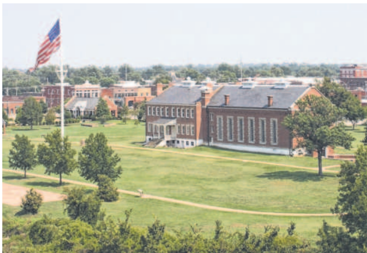
FORT SMITH NATIONAL HISTORIC SITE
